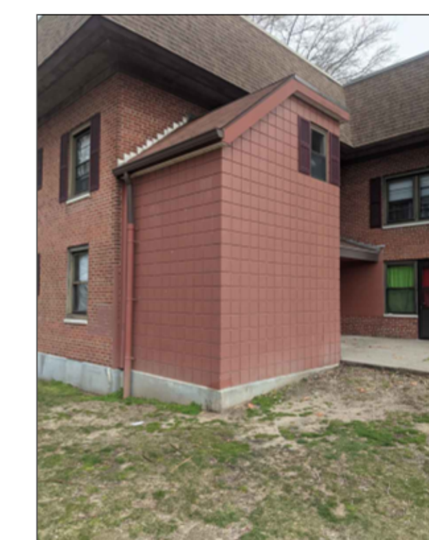
TYPICAL REAR VIEW OF STAIR TOWER
