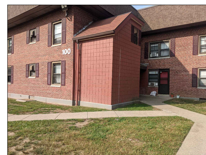
TYPICAL VIEW OF STAIR TOWER 100A
