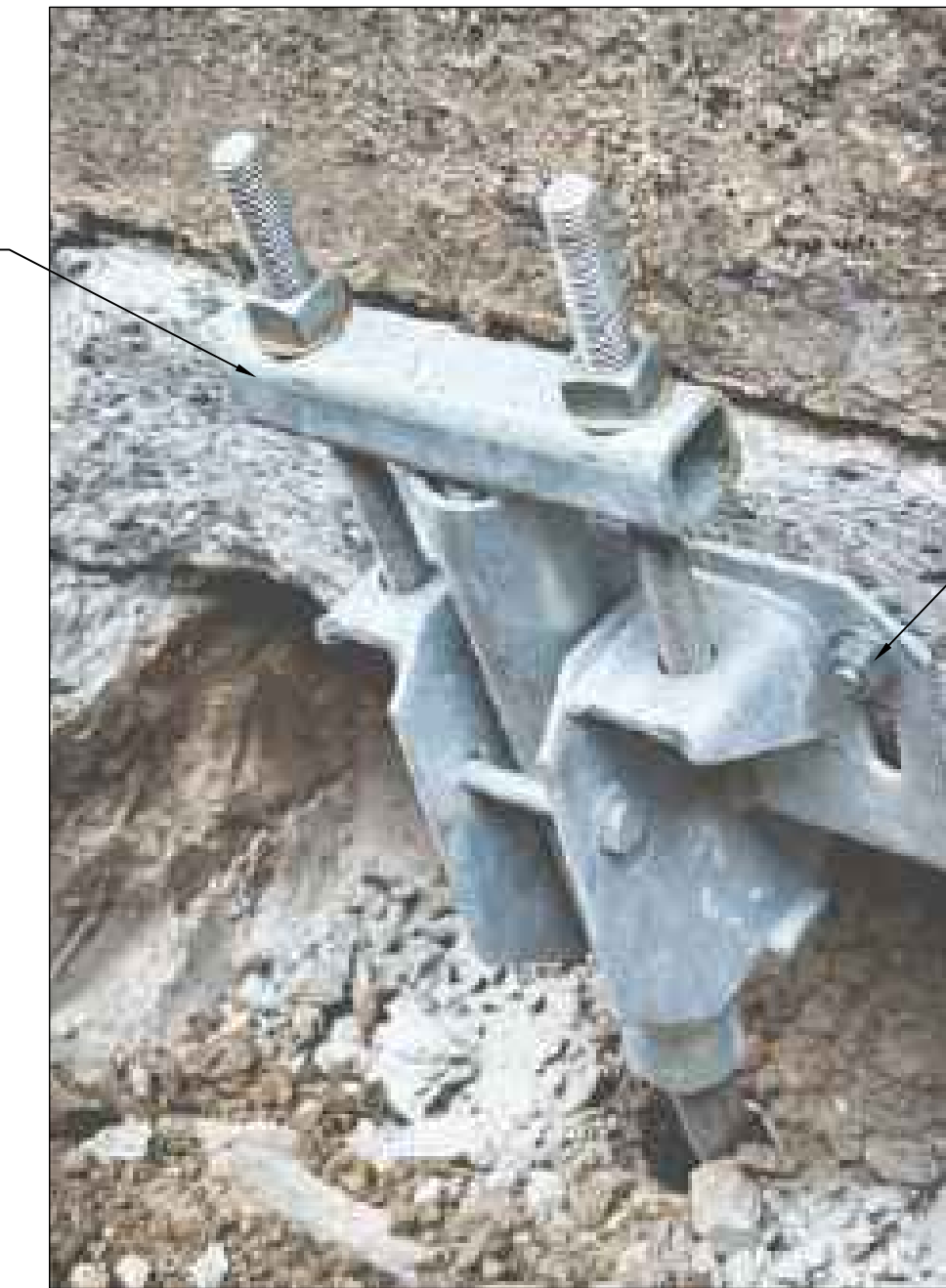
TYPICAL HELICAL PILE MOUNTING BRACKET
